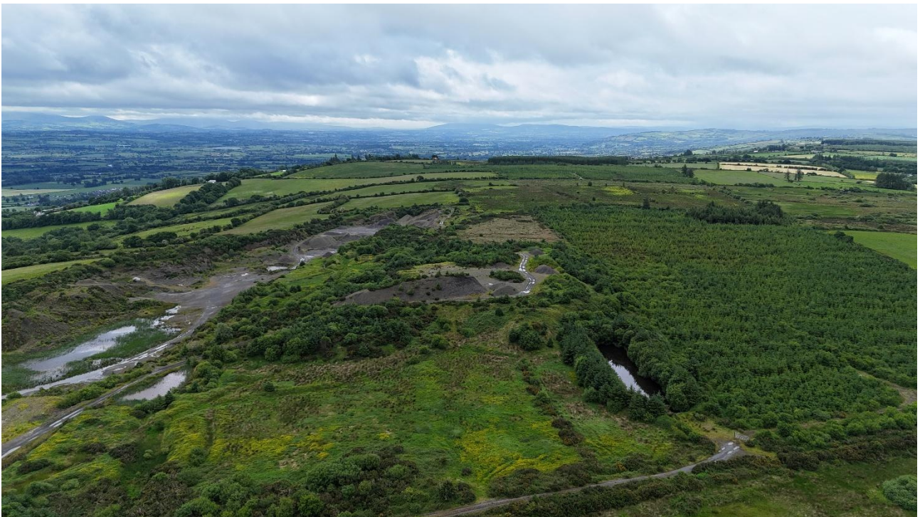
Plate 14-2: Drone view of area 2 looking south.
